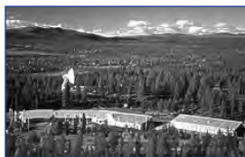
Figure 10-3 ESA operates several ground stations, including this Kiruna S-band and X-band station in Sweden.
