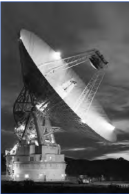
Figure 1-7 The 70 m Goldstone radar near Barstow, CA is capable of detecting 2 mm objects in LEO.
